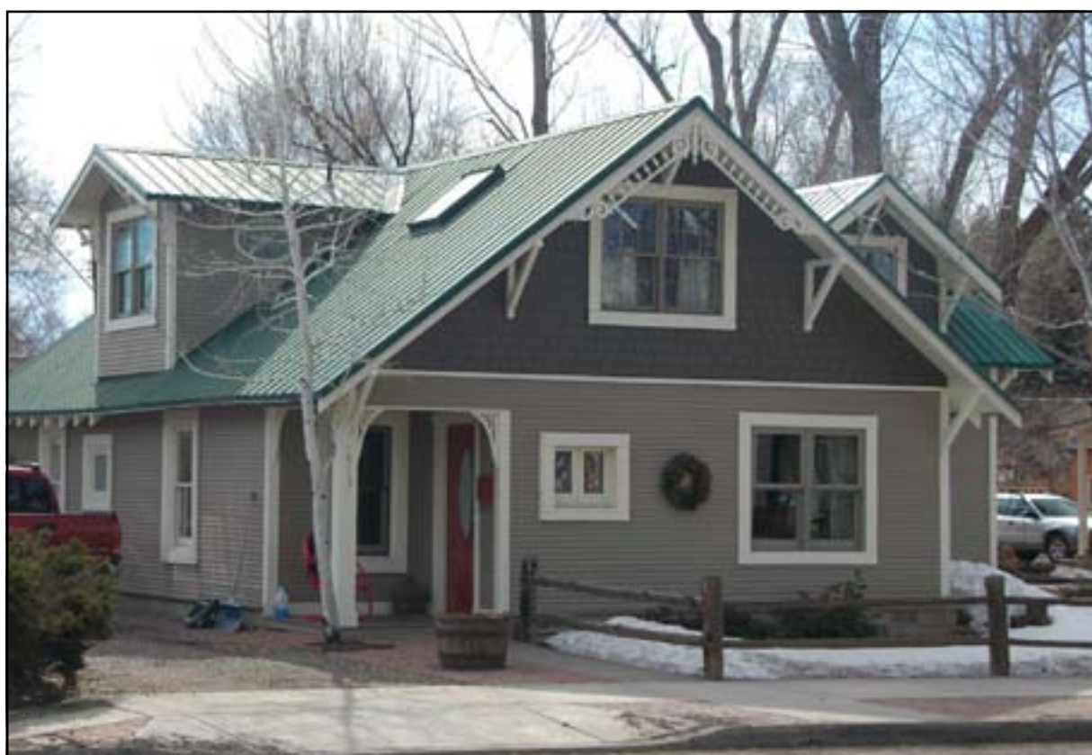
A single-family house with a recessed stoop.
