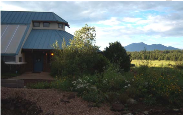
Photo 15: Building at Arboretum of Flagstaff, is reflective of the landscape in scale and materials.. Photo by Deborah Soltesz, 2010.
