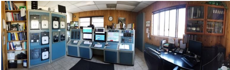
The 60-year-old analog system filled the room and used paper charts to record data.
