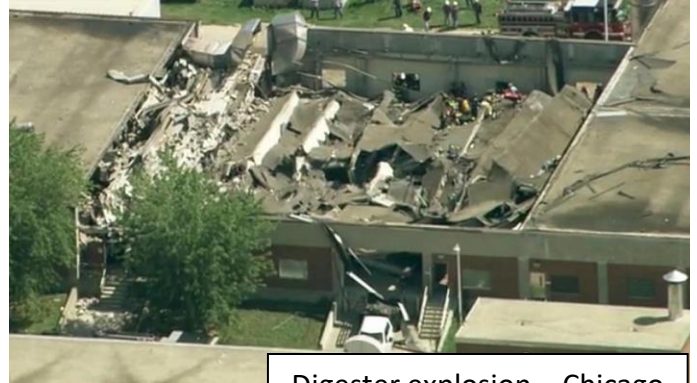
Digester explosion – Chicago Tribune, August 2018
