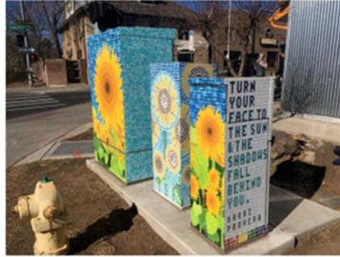
Traffic signal cabinets are the stainless-steel structures located at every signalized intersection. Artist designs can be printed on 3-m patented vinyl, which is easily maintained, is removable, and has been demonstrated as safe technology to use on signal and utility cabinets. A vendor will be solicited separately for the production and application of the vinyl wraps. Above are examples of two sites completed last year as part of a pilot project.
