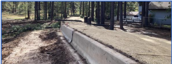
Reinforced Concrete Barriers on Backfilled Berm
